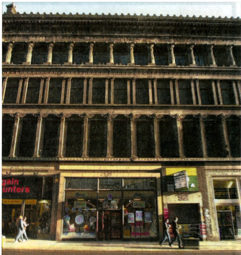
UNDER THREAT: Alexander "Greek" Thomson's historic Egyptian Halls in Glasgow.
