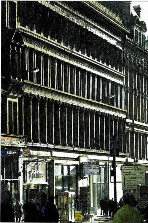
THREAT: The facade of the Egyptian Halls on Glasgow's Union Street. Its
